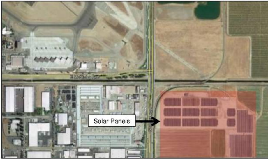
Figure 22 Solar panels at Fresno Yosemite International Airport
