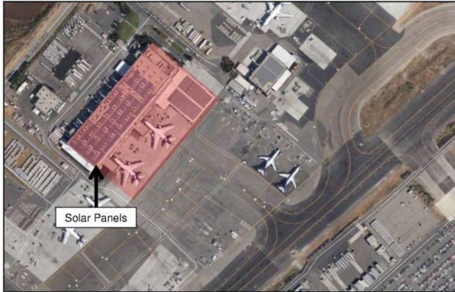
Figure 24 Solar panels at Oakland International Airport
