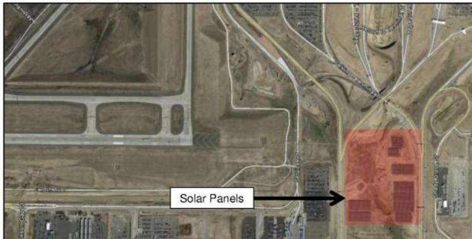
Figure 21 Solar panels at Denver International Airport
