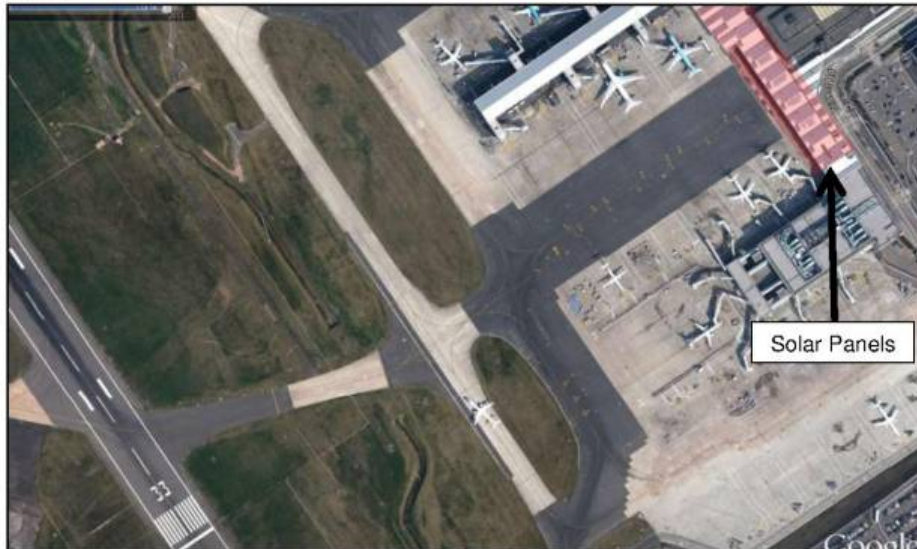
Figure 19 Solar panels at Birmingham Airport
